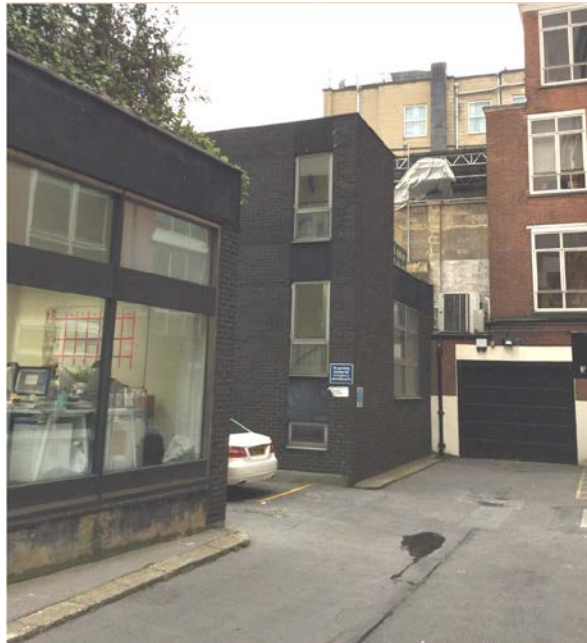
Existing view from Grantham Place
